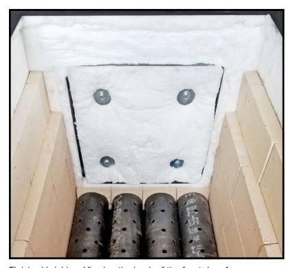
Finished bricking. Viewing the back of the front door frame. NOTE: This photo is shown WITHOUT Smoky Lake Brick Batter (High Temp Mortar)
