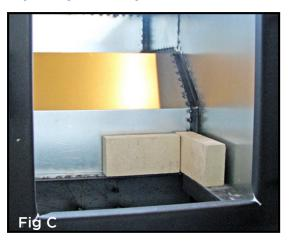
This photo, looking through the door of the firebox, shows the ledge upon which your first layer of bricks will sit. NOTE: Ceramic blanket will have been installed by this point even though these photos don't show it.
