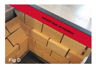
The space blocked in red represents the long skinny strip of insulation described in step 6 above. This second layer of insulation should pack snuggly between the top arch rail and the top brick layer. Do the same thing on the left side of the firebox.
