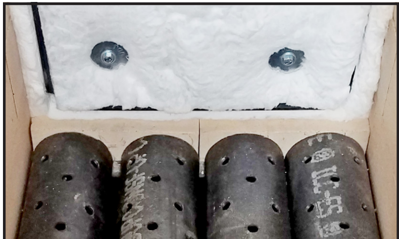
Finished bricking. View of Bricks E under the door. The upgraded Domed Cast Iron grates are also shown in place. NOTE: This photo is shown WITHOUT Smoky Lake Brick Batter (High Temp Mortar)
