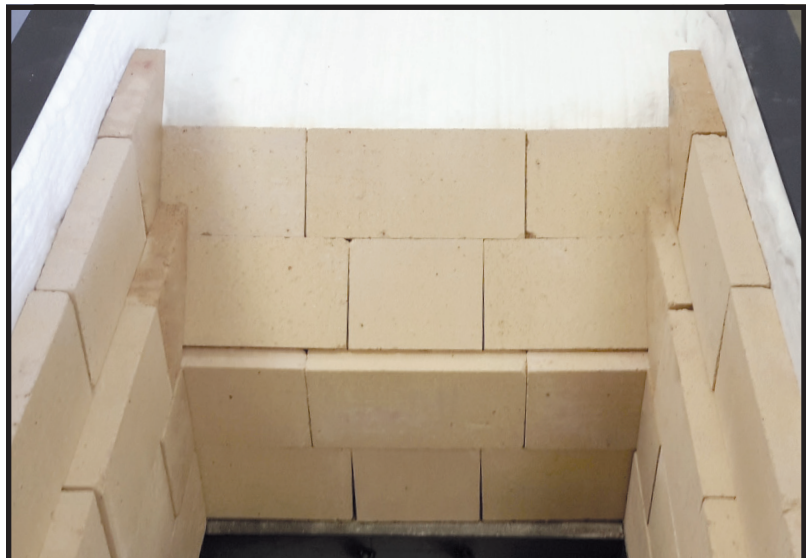
Finished bricking. View of the back wall and ramp of the firebox. NOTE: This photo is shown WITHOUT Smoky Lake Brick Batter (High Temp Mortar)
