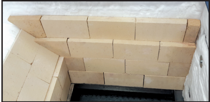
Finished bricking. View of the right side wall inside the firebox. NOTE: This photo is shown WITHOUT Smoky Lake Brick Batter (High Temp Mortar)
