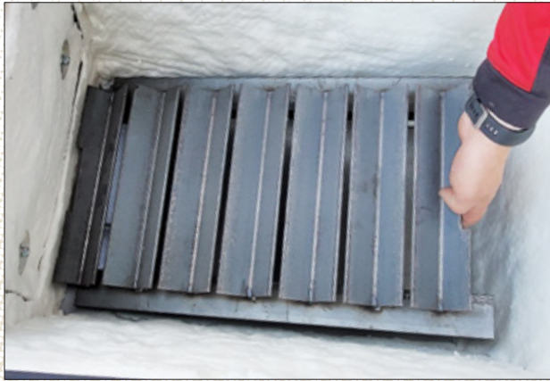
Fig 7J — The end of the grate assembly in which the base extends past the “Vs” should be positioned at the back of the Firebox.
