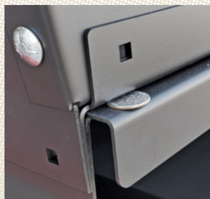
Fig 4B Use dime spacers in the front
